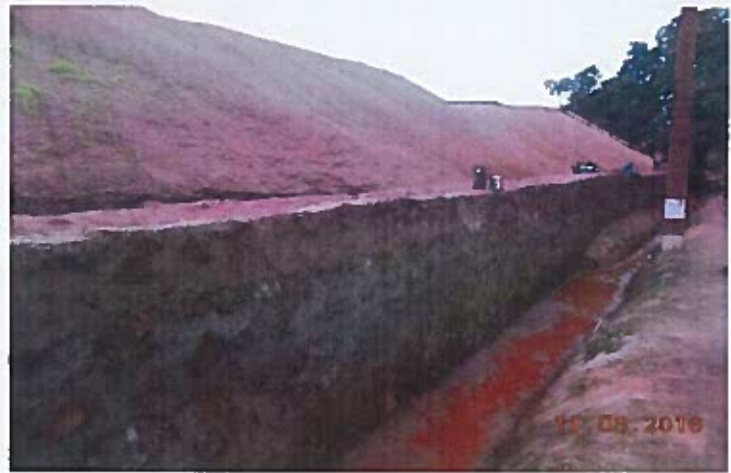
DUMP WITH RETAINING WALL, GARLAND DRAIN
