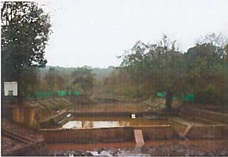
CHECK DAM FOR NALLAH PROTECTION
